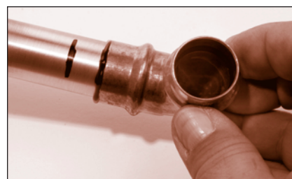
FIGURE 89: Visual check of adhesive coverage
