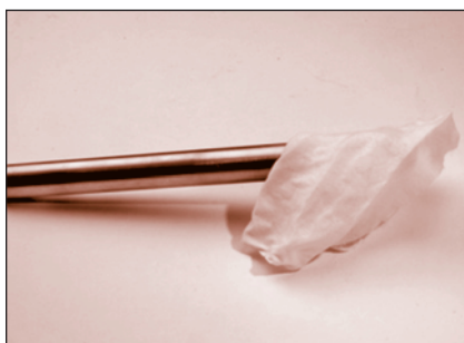
FIGURE 84: Wipe with premoistened alcohol wipe or pad
