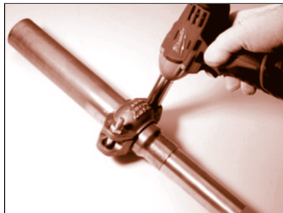
FIGURE 43: Tightening the clamp
