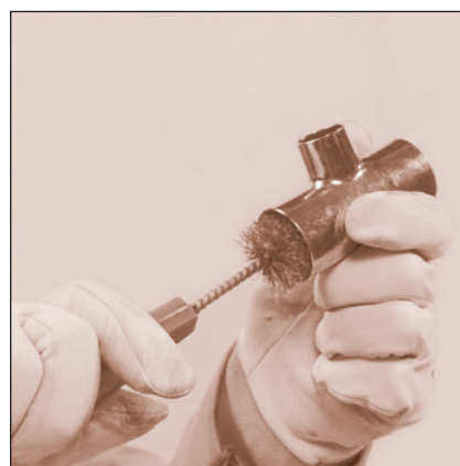
FIGURE 17: Cleaning: Fitting brush
